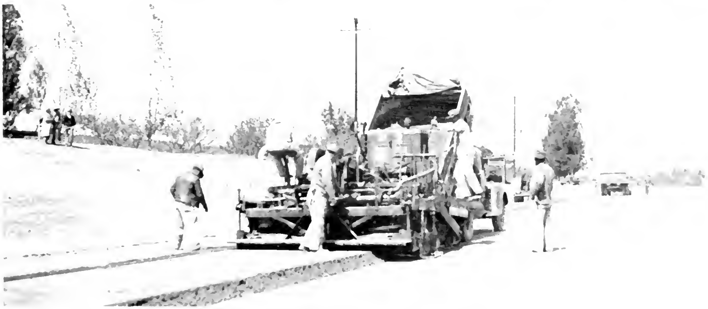
Spreading cement-treated base material with self-propelled mechanical spreading machine which pushes truck discharging material ahead of it
